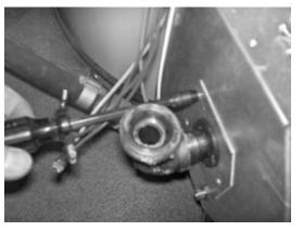
Step 6: Remove pipe flange plate from Burner Box
